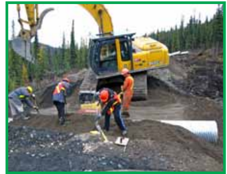
Construction of a cross drain.
