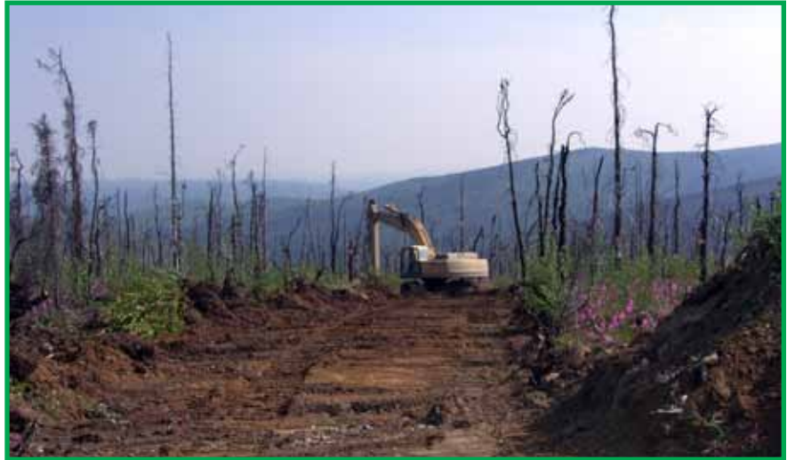
Trails and roads should not be constructed wider than required to bring equipment safely to site.
