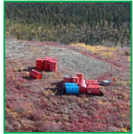
Example of a small fuel cache located a safe distance from any watercourse. Note signage indicating type of fuel (orange picket with sign attached), spill kit (grey and green plastic container located left of sign) and full drums are placed in a portable berm.
