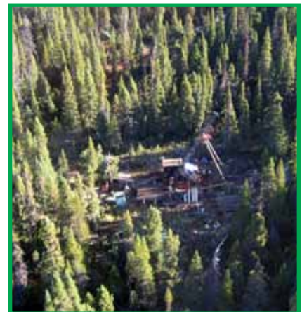
Keep clearings and the removal of vegetative mat for drill pads and trails to a minimum.
