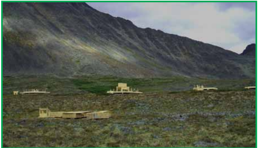
Well planned temporary closure. Note core boxes and wood is neatly stacked, tent canvas has been removed from tent frames, and all plastic and metal has been removed from site.
