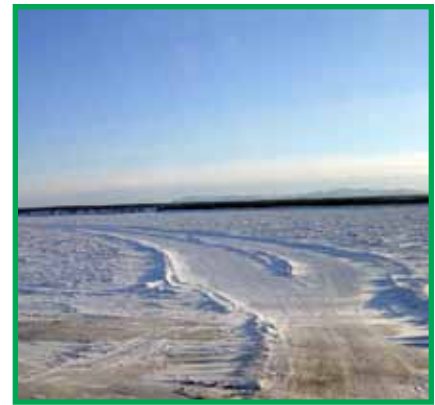
The approach area for winter road crossings on lakes or streams should not be steep and cutting riparian vegetation should be kept to a minimum.
