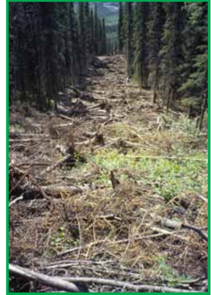
Reclaimed trench. Note branches and other organic material scattered over the site to promote natural revegetation.
