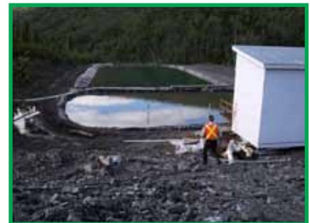
Advanced projects require infrastructure such as water treatment plants, settling ponds etc. If the project does not proceed the infrastructure will have to be removed and the disturbed areas reclaimed.
