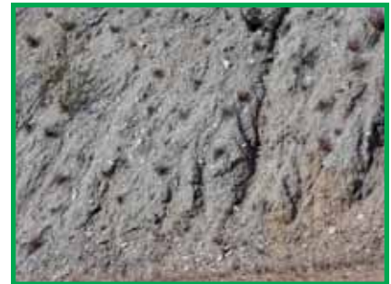
Improper reclamation will cause erosion to occur. Note: rills and gully erosion occurs when ground has not been recontoured properly.
